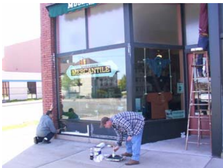
The Muskegon Mercantile storefront gets a fresh coat of paint.
